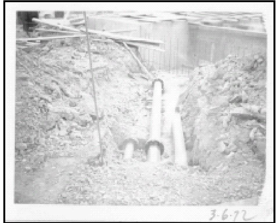
**Photo 12** - March 6, 1972 photo. View looking southwest toward the northeast corner of the EQ tank. The three pipes are presumed to be from Bldg 2 WW tank area. Rebar from Neutralization tank wall construction in background.
