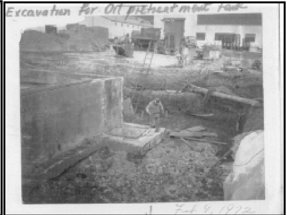
**Photo 6** - February 9, 1972 photo. View looking northeast from near north mandoor of WWTP building. Note former sump pad and excavation for new EQ tank.
