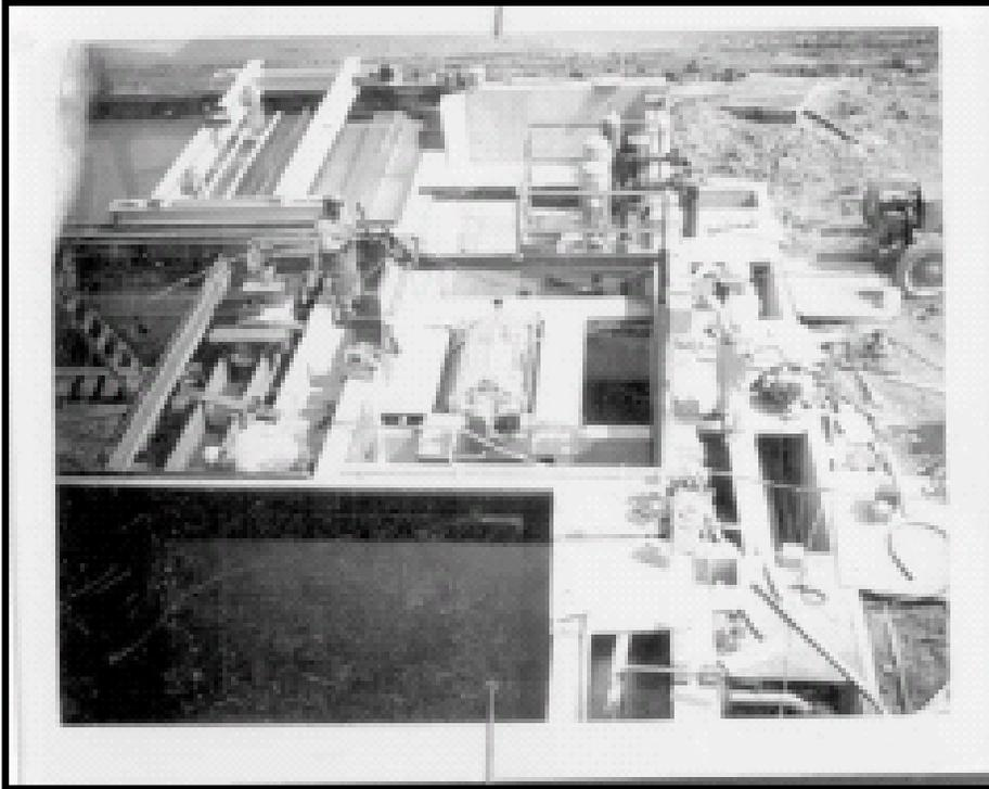
**Photo 21** – Undated photo. View looking north from WWTP roof at new Microscreen installation. Pipe trench is present along east side of tanks and is partially covered and north settling basin is full.
