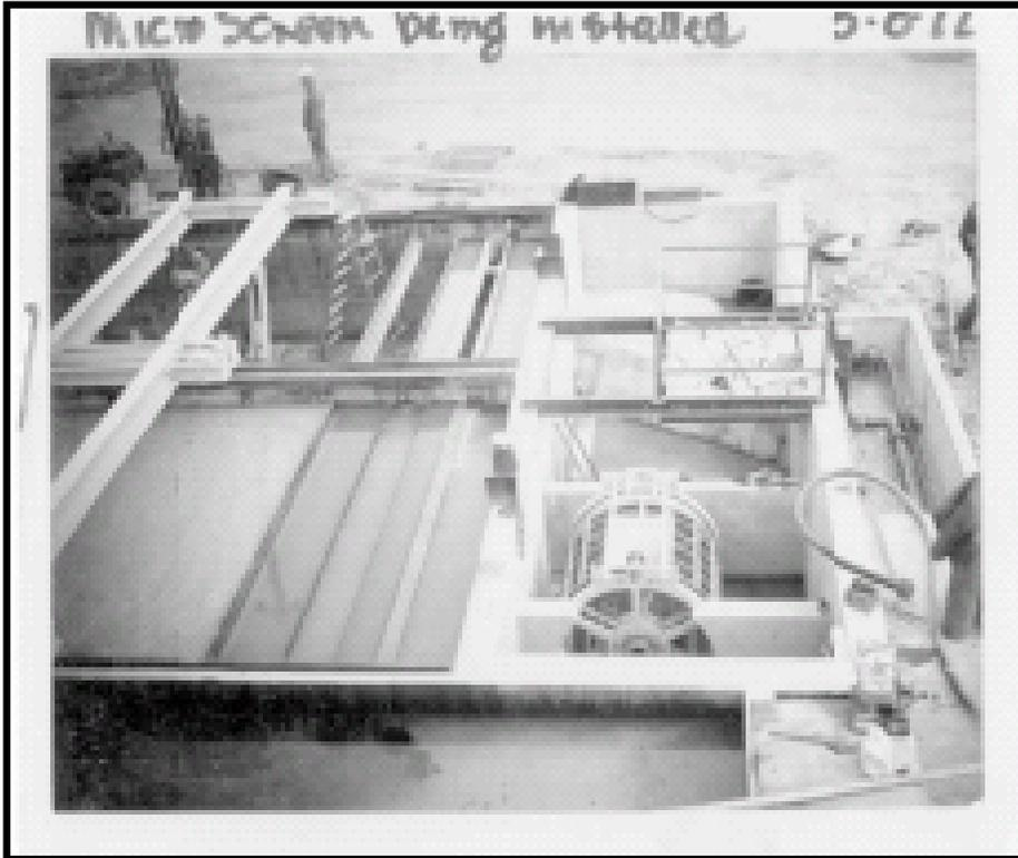
**Photo 19** – May 8, 1972 photo. View looking northwest from WWTP roof at new Micro screen and effluent discharge point (northeast corner of Oxidation tank). Pipe trench is present on the right-hand side.
